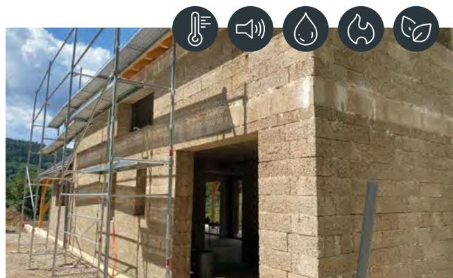
**Project:** Construction of a single-family house with the Hempro system made of 36cm hemp blocks. The owners were convinced of the advantages of a single-wall system and wanted to use bio-based products as much as possible. Building with hemp blocks was therefore the most logical choice.
