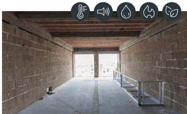
**Project:** For the interior renovation of a former two-story office building, 15 and 30 cm hemp blocks were used to transform the building into 9 lofts that meet very low energy standards. The entire inner shell was made of hemp blocks which were also used for the double partition walls. Result: optimal sound insulation and fire-resistant walls. The natural interior plaster of IsoHemp was also used as a filler layer for interior walls.
