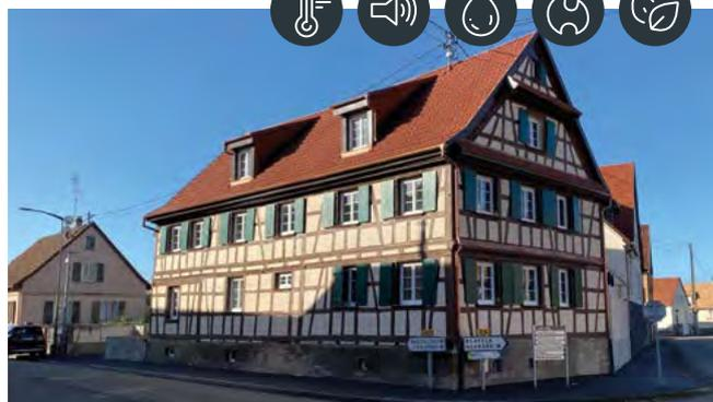
**Project:** The heritage of the Alsace region is of great historical value and must be preserved. The renovation of a half-timbered house is a technical challenge where many parameters must be taken into account, including thermal insulation and moisture regulation so as not to damage the wooden framework. In this case, hemp block are the obvious solution, as it stays close to the know-how of the past.
