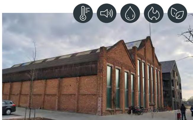
**Project:** Construction of 8 storage rooms for the preservation of works of art of the city of Mechelen. This project has a “box in a box” structure with walls of 30cm thick blocks and between 6m and 8m high. A total of 1500m<sup>2</sup> of hemp blocks were used.
