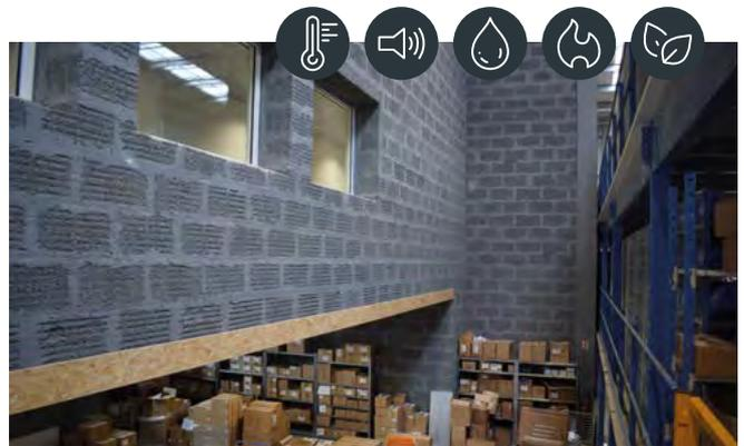
**Project:** New industrial building constructed from 30cm thick hemp blocks and a supporting structure of concrete blocks. The building includes a logistics centre and various office spaces.
