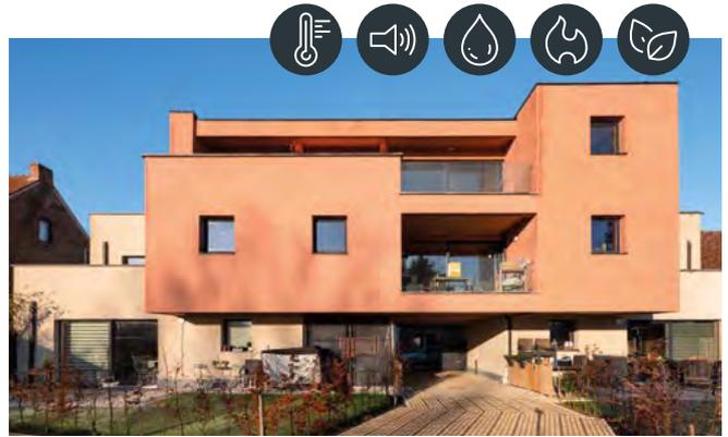
**Project:** A new apartment building built with CLT and an outer shell of 30 cm thick hemp blocks. The client was looking for natural and breathable insulation. The interior walls consist entirely of 12 cm thick hemp blocks that significantly improve the acoustics of the living spaces.
