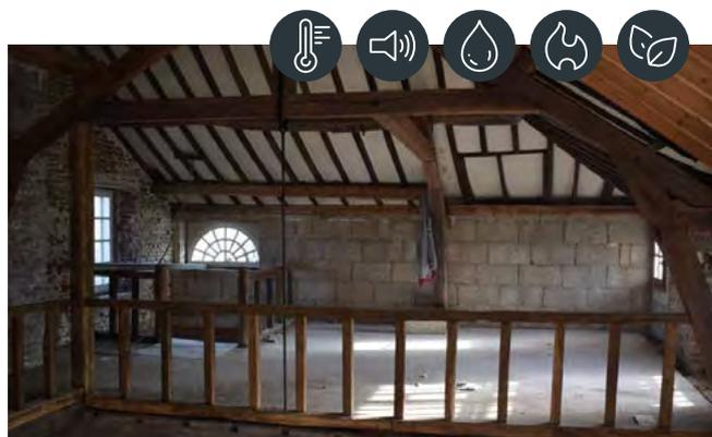
**Project:** Complete interior renovation of an old barn using 15 cm thick hemp blocks. The aesthetic character both on the inside and on the outside of the former farmstead is preserved, and potential condensation problems are avoided, thus leaving the wooden roof unaffected. Along the inside finished with natural plaster based on lime.
