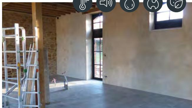
**Project:** Renovation and restoration of the inside of a former French 'longère' (longhouse farm, which in this case served as a pig farm) using 20cm hemp blocks. Preserving the external character of the building with old authentic stones. Plastered on the inside with lime.
